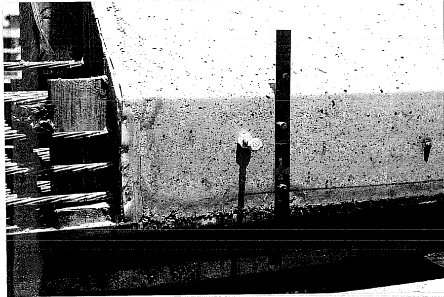
a) view of bottom flange at the south end of L-I2
